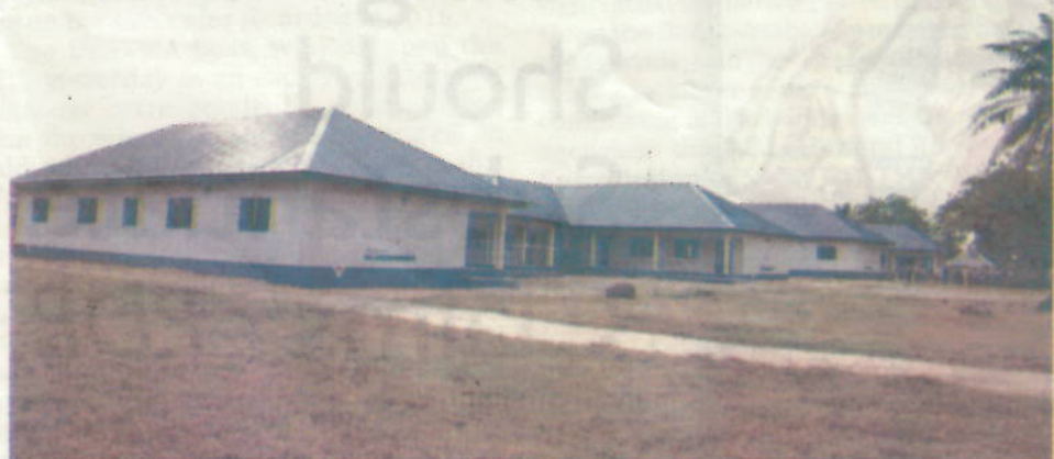
A Cross Section of the newly built 12 classroom blocks at Utagba-Ogbe Grammar School, Kwale, Delta State.
